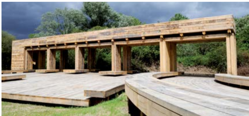
Observatorium, Péage Sauvage © B. Renoux/LVAN
